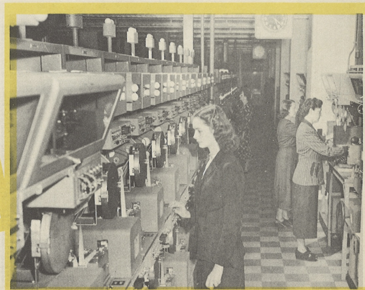
At telegraph message center, electrical equipment automatically speeds the message to destination.
